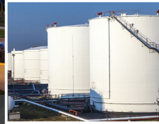
Storage Tank Farms
